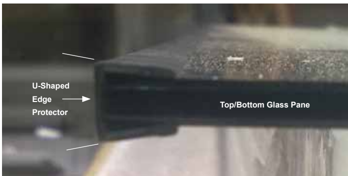
Figure 6B.2 - Outer Glass Edge Protector
