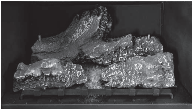
7. Using the brush supplied, lightly brush the ember wool onto the Centre of the burner & in between the logs on the left and right. try not to have heavy clumps of wool.
