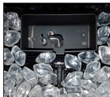
Figure 16. Ignitor assembly beside the burner.
