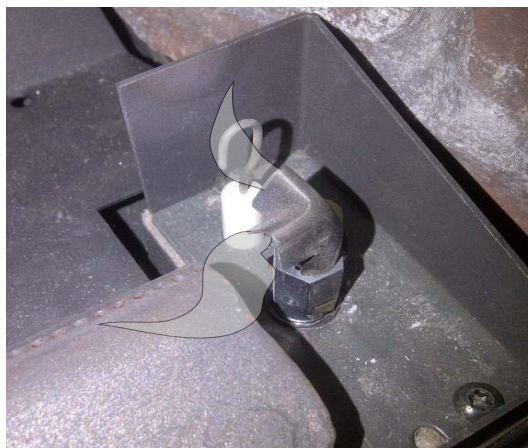
Figure 22: Correct Pilot and Pilot Shield Orientation
