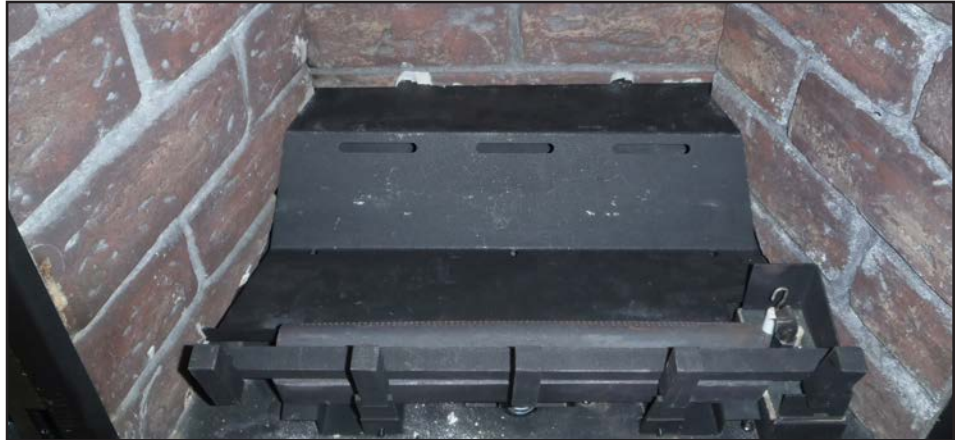
Figure 58: Empty firebox with grate and locator pins.
