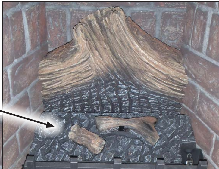
Figure 59: Back Log and Ember Bed Installation.
