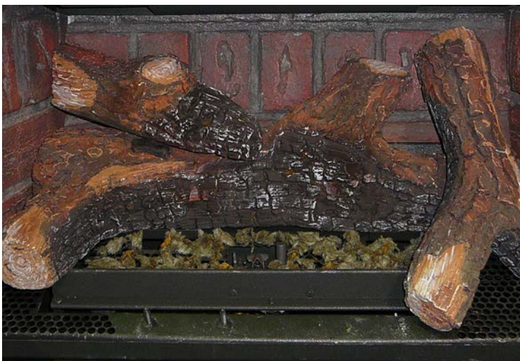
Figure 64: Fifth Stage Log Set Installation.
