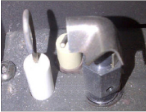
Figure 19: Proper Pilot Position
