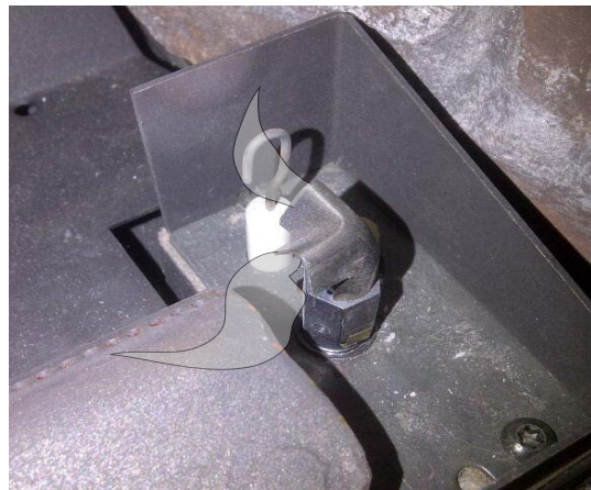
Figure 23: Correct Pilot and Pilot Shield Orientation
