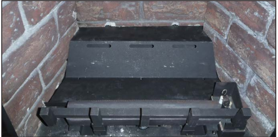
Figure 45: Empty firebox with grate and locator pins.
