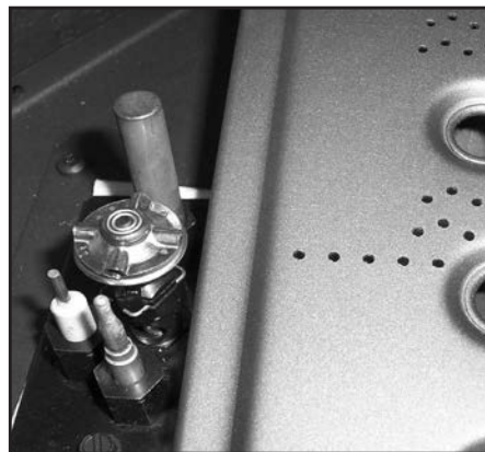
Figure 15: Ignitor assembly beside the burner.
