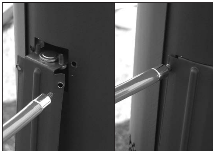
Figure 48: Spill switch installation.
