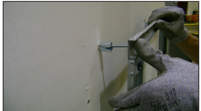
Figure 5 Installing Anchors in Hollow Wall
