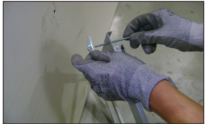
Figure 4 Toggle Bolt Installation through Mounting Bracket
