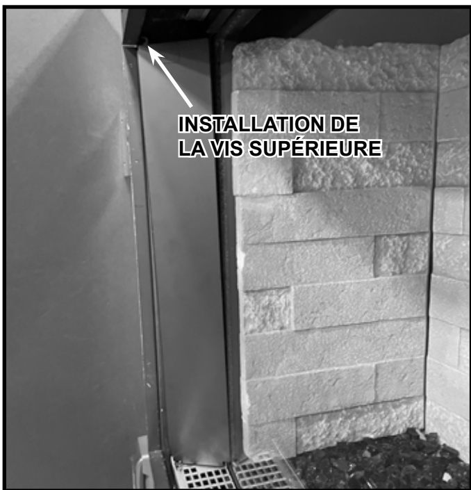
Figure 4.11 Panneau de transition installé
