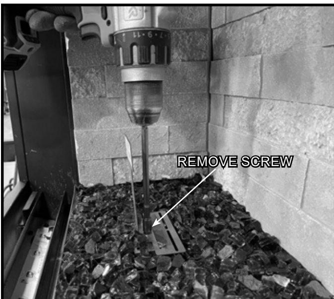
Figure 11.4 Place Media, Remove Media Placement Jig Screw
