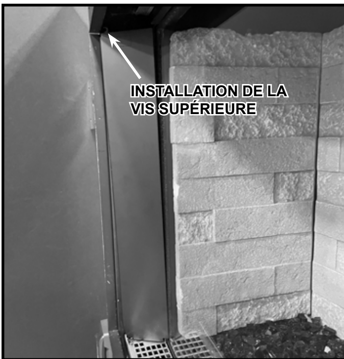
Figure 11.21 Panneau de transition installé
