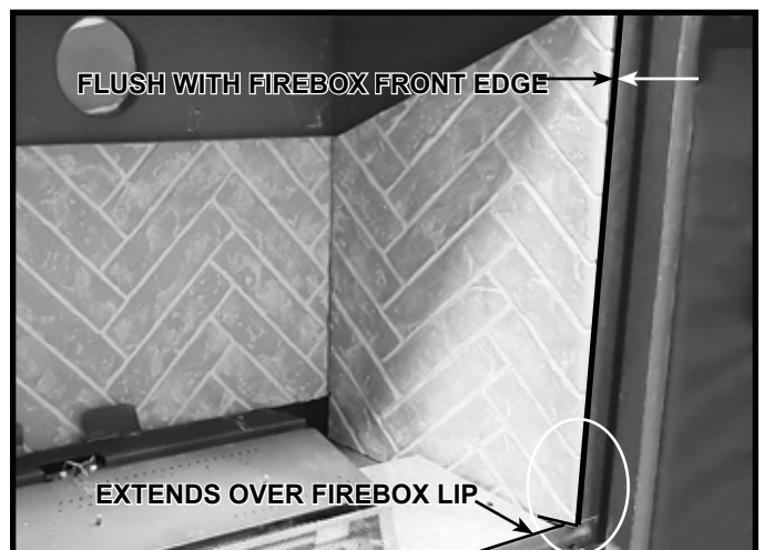
Figure 11.4 Side Refractory Panel Installed (Right Side Shown)
