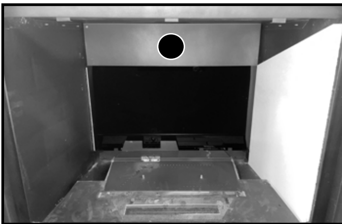
Figure 11.17 Rear Glass Panel and Side Insulation Board Installed
