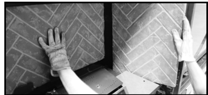
Figure 11.3 Install Side Refractory Panel (Right Side Shown)
