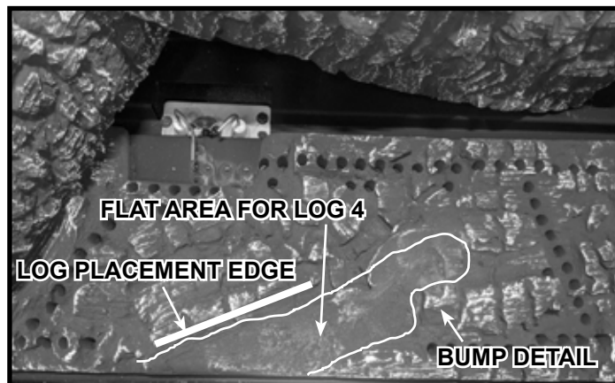
Figure 8 Log Placement Details
