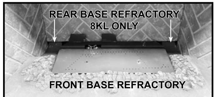
Figure 11.8 Base Refractory Pieces Installed
