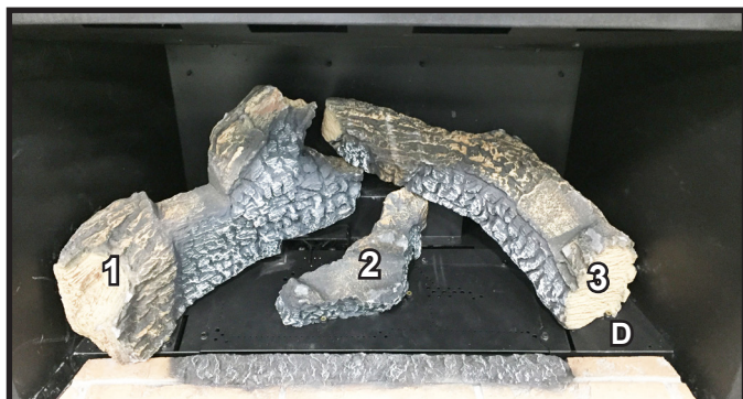
Figure 14. Bûche n° 3 installée
