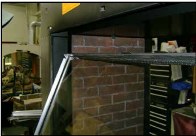
Figure 11.2 Initial Positioning of Frame into Opening.
