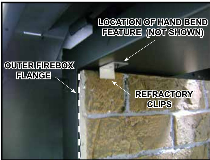
Figure 11.16 Refractory Clip Installation
