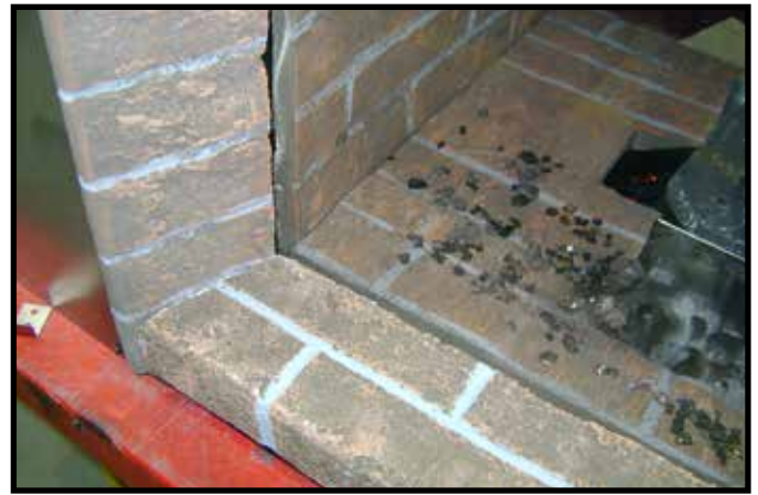
Figure 11.28 Outer Hearth Installation
