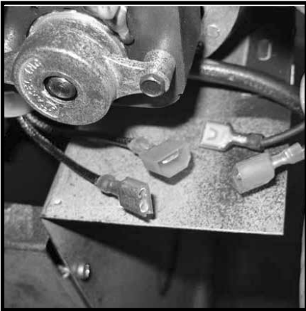
Figure 15: Disconnecting fan wires.
