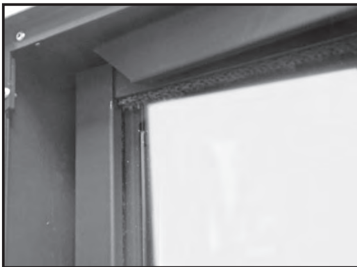
Figure 66: Installing top trim.
