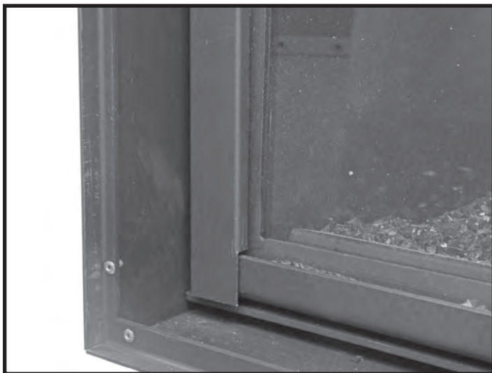
Figure 65: Side trim in place.
