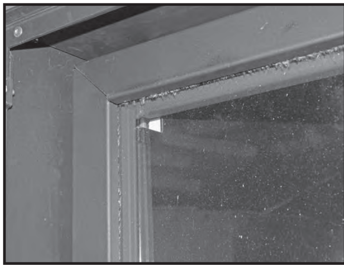
Figure 67: Top trim in place.
