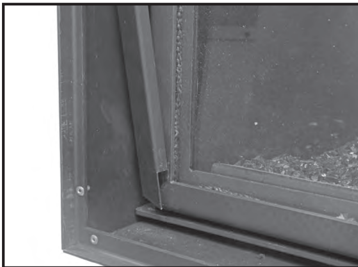
Figure 64: Installing the side trim.
